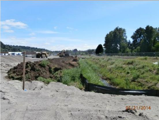
***Realignment of drainage channel along Dike Access Rd.***
